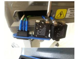
Transfer wire terminals one at a time from old Circuit Breaker to new using #2 Phillips Screwdriver, noting terminal connections and circuit breaker orientation are correct as shown
